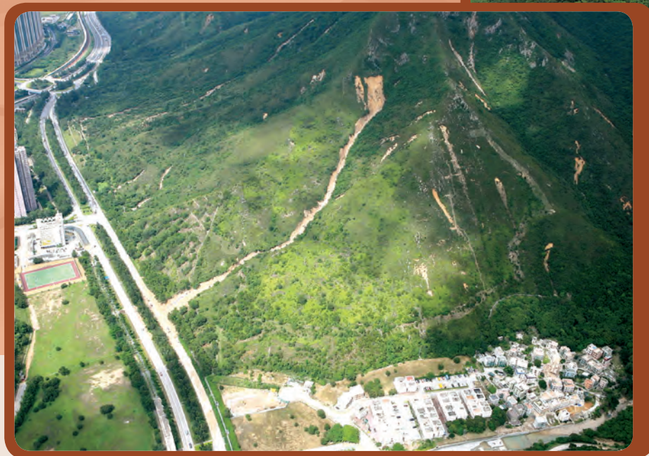
2008年裕東路天然山坡山泥傾瀉，導致西行線被封閉4天 Yu Tung Road Natural Terrain Landslide in 2008, resulting in closure of westbound traffic lanes for 4 days
