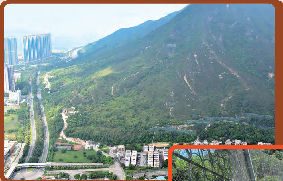
東涌壩尾的天然山坡山泥傾瀉災害緩減措施（柔性防護網） Natural terrain landslide hazard mitigation measures in Pa Mei, Tung Chung (flexible barrier)
