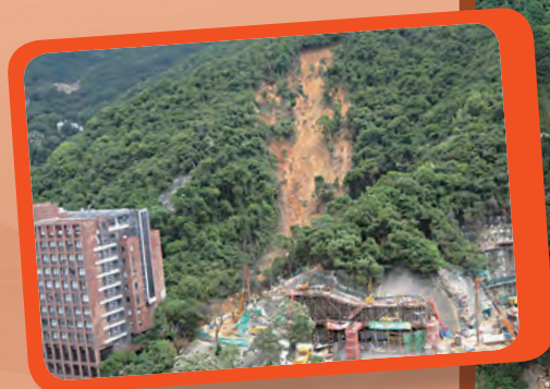
2008年香港大學天然山坡山泥傾瀉，導致周亦卿樓部分樓層受損 University of Hong Kong Natural Terrain Landslide in 2008, resulting in damage to several floors of Chow Yei Ching Building
