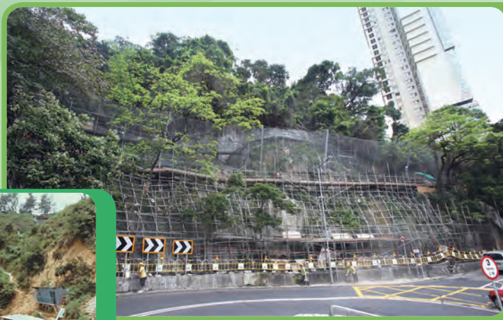
鞏固不合標準斜坡 Upgrading substandard slopes
